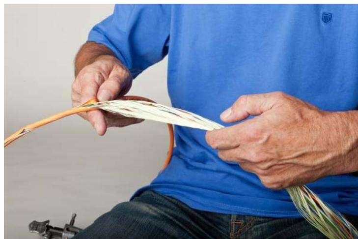
7. Cut the central strength element and use the appropriate scissors to remove aramid or glass yarns
