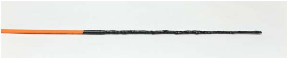
Fix the cable to the pulling rope / tape using a specially designed pulling grip for optical fibre cable (length of 600mm minimum) to ensure that the pulling tension is well distributed on all cable components (outer sheath and reinforcing elements).
